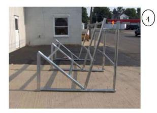
After the BK-4's are bolted into the center upright it is time to bolt the BK-0's on the back ramp portion of the upright section.
