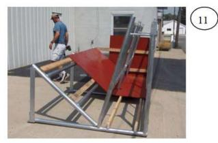
Put in the floor section. This runs from the ramp to the front upright pipes.
