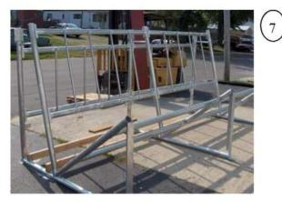
With the frame bolts tight put in the floor boards. It is best to use 2" x 4" x 12' and cut them down to span two sections at a time.
