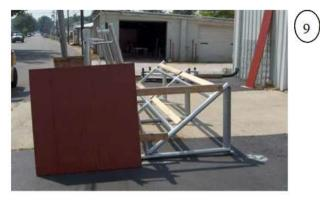
Put the 2" x 4"s on the ends along with whatever you are going to cover it with. Here we are using a half sheet of plywood.
