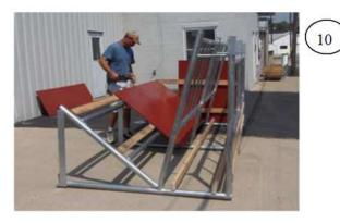
Put on the ramp. If you are using plywood use a full 4' x 8' sheet so it spans over to the next 6' of the feeder creating even more strength.
